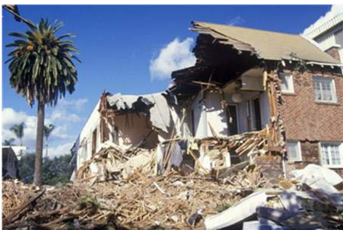
Damage from the 1994 Northridge earthquake
